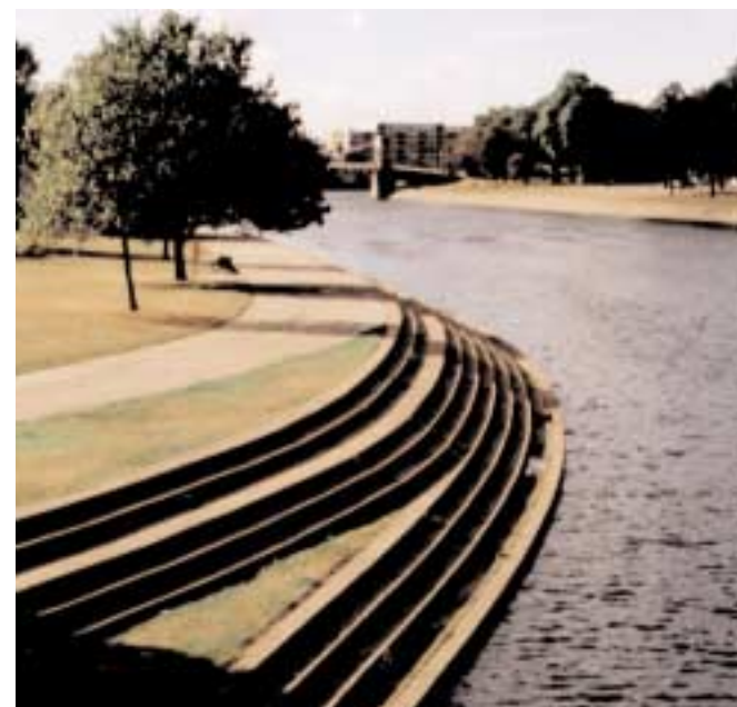
Figure 1.75 The River Trent at Trent Bridge in Nottingham where it has been widened and lined with concrete.
