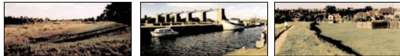
Figure 1.76 Channelisation of the River Trent in Nottingham has reduced the risk from flooding.
